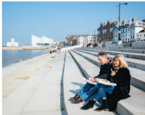
Margate Flood Defences
